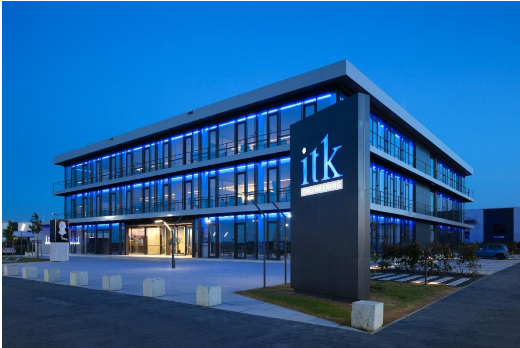
ITK headquarters in Rülzheim, Germany. (Photo credit: Nikolay Kazakov)
